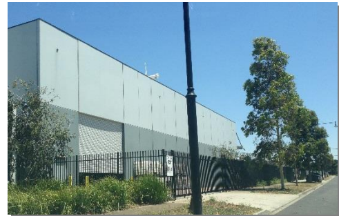
Two tone facade to disguise the blank walls facing street boundary. Suitable fencing demonstrated. ( above right )
